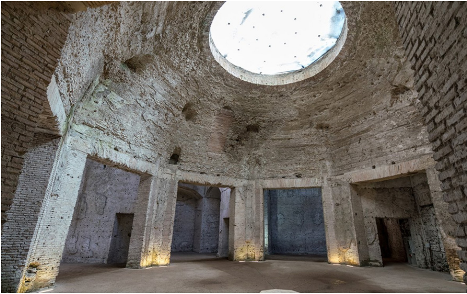
Fig. 1. Octagonal domed hall in the centre of the Domus Aurea ( Fototeca Unione ).
